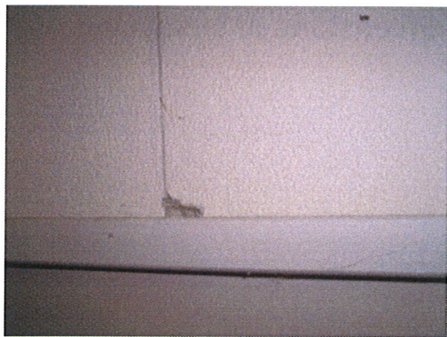
Figure 4 – Phone Room Ceiling (Sample 4) ceiling flat sheet Area: 12 m 2
