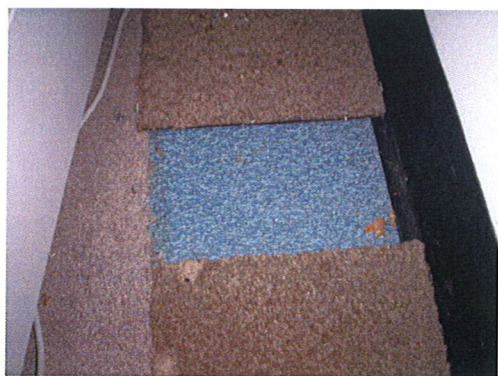
Figure 10 – Mermaid room/staff room under carpet (Sample.10) Vinyl floor covering Approx Area: 180 m 2
