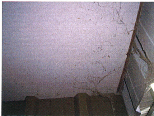
Figure 1- Woodbox entry alcove (Sample 1) Internal ceiling flat sheet Area: 3m 2
